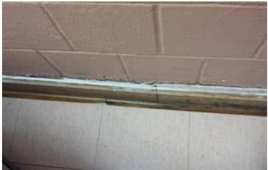
Damaged Floor Board and Black Mold
