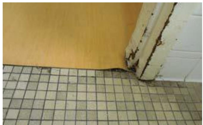
Damaged Rusty Doorway, Black Mold on Floor,
