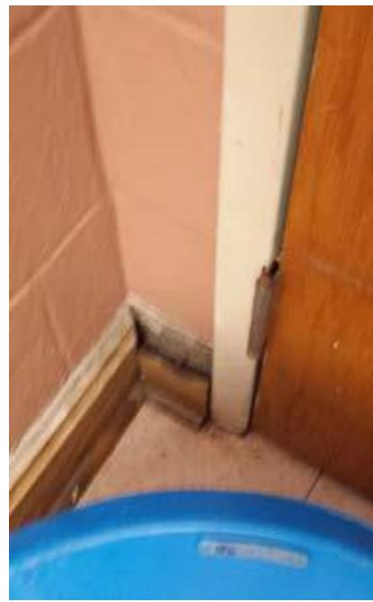
Missing Floor Board and Black Mold
