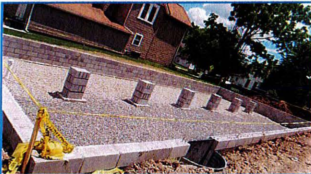
A firm foundation awaits the home. No local dollars were spent on the land due to the availability of federal funds.
